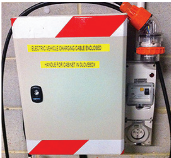
DOT three-phase outlets
