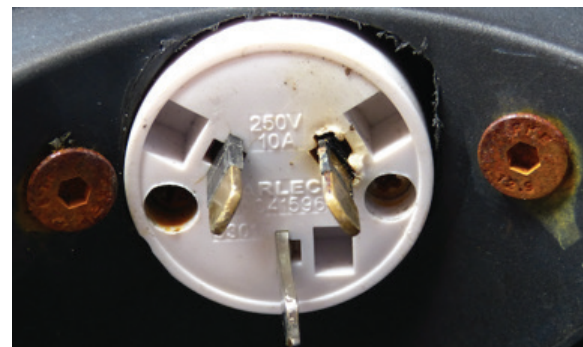
Original single-phase vehicle inlet with burn marks
